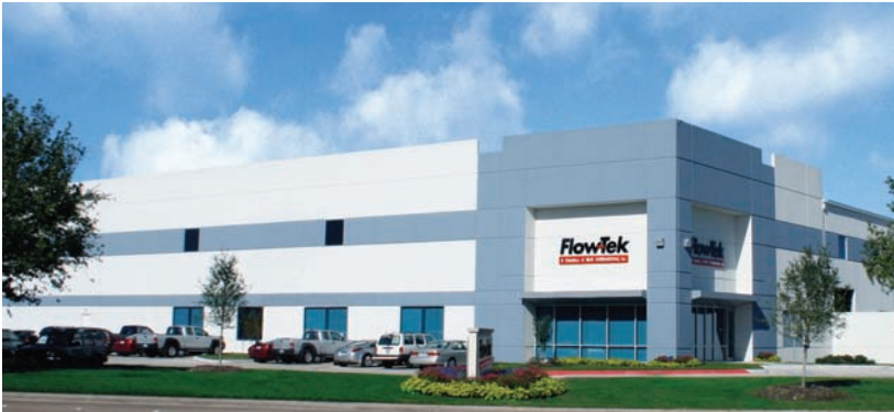
Flow-Tek, Inc. – headquarters, Houston, Texas
